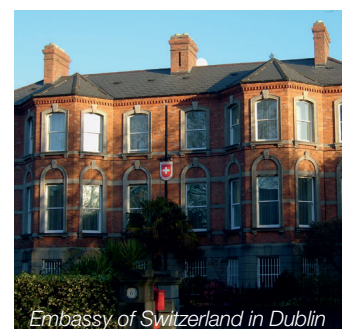
Embassy of Switzerland in Dublin
