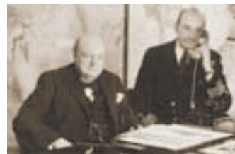
In the bunker: Churchill directing the war from underground headquarters.
