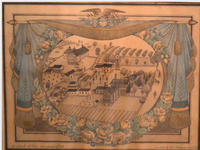
Portage County Infirmary by Ferdinand A. Brader (1833-1901). Graphite and colored pencil on wove paper, 22 x 28 inches. Courtesy of the Portage County Historical Society, Ravenna, Ohio. Brader stayed at the Portage County Infirmary, commonly known as the "poor house" from 12 December 1891 until 19 April 1892. The following four years until his return to Switzerland in February 1896, he stayed at the Stark County Infirmary, Canton, Ohio
